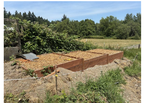
A Denitrifying Bioreactor (above) uses carbon to manage nitrogen
